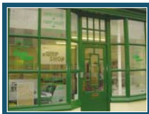
The Swap Shop after refurbishment
